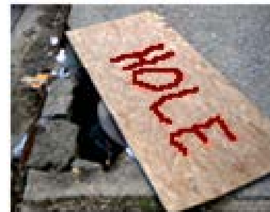
Figure 9. Plywood hole cover.
