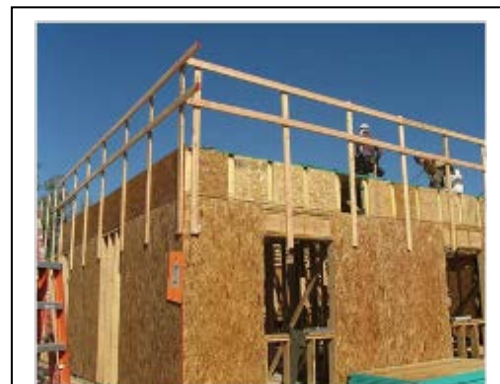
Figure 4. Temporary guardrails.
